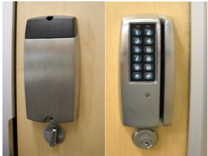
Figure 1. Photos of Electronic Lock Assembly: Inside and Outside Views
